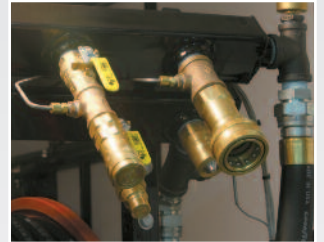
Electronic temperature monitor at H.T.F returns.
